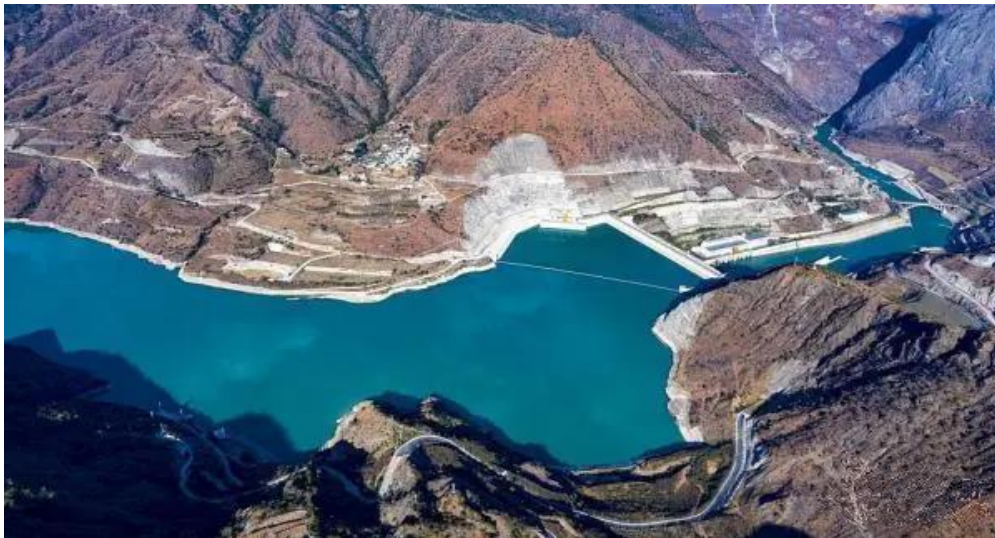
Birdview of Liyuan Dam and Reservoir
